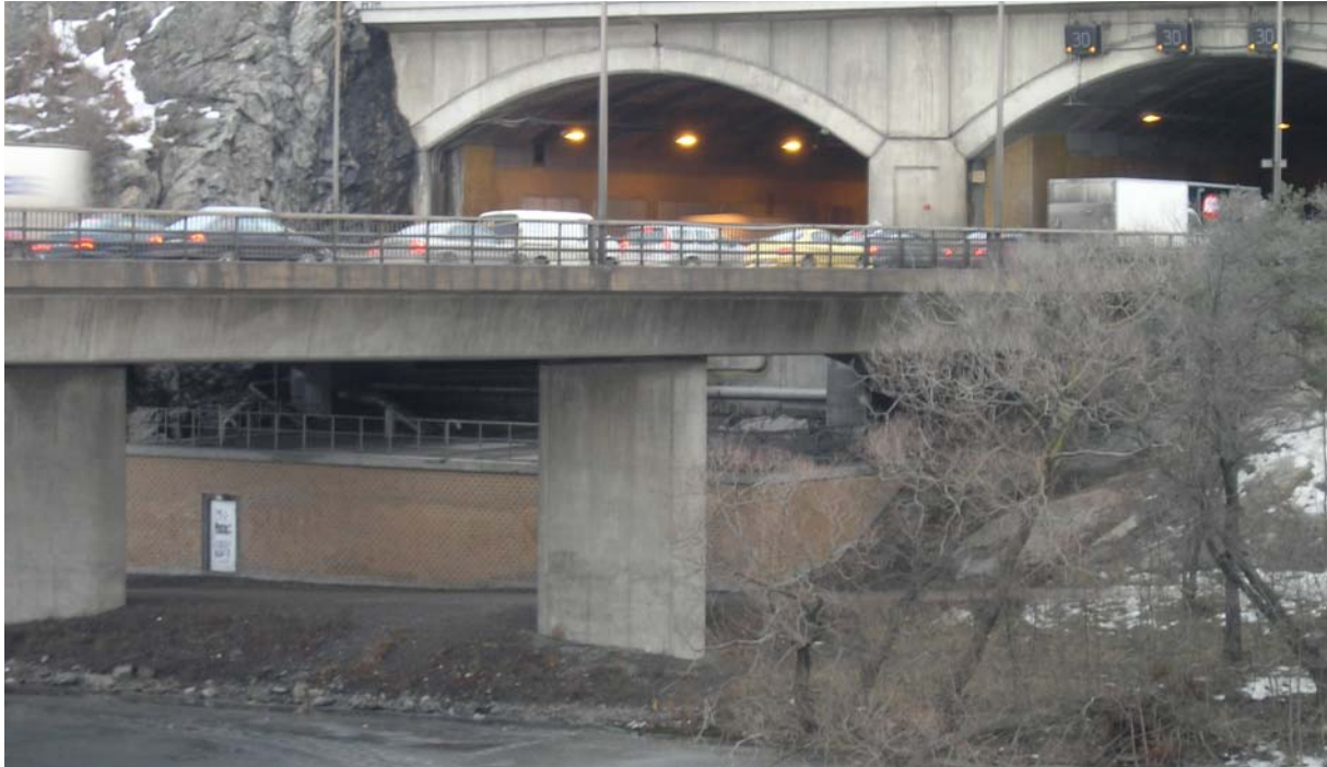
Figure 9 Fredhäll treatment plant for stormwater
