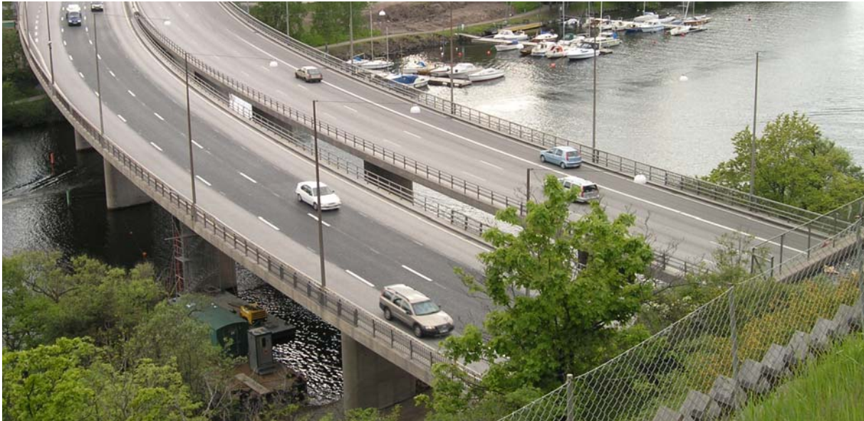
Figure 10 Fredhäll catchment area (north bound traffic in left lane)
